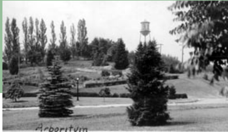
Arboretum with "T" tank in background. University of Idaho.
