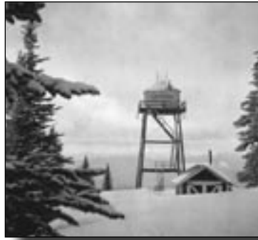
Looking Glass Lookout, circa 1940. Renamed Gisborne Lookout in 1949 and dedicated as such in 1951.
