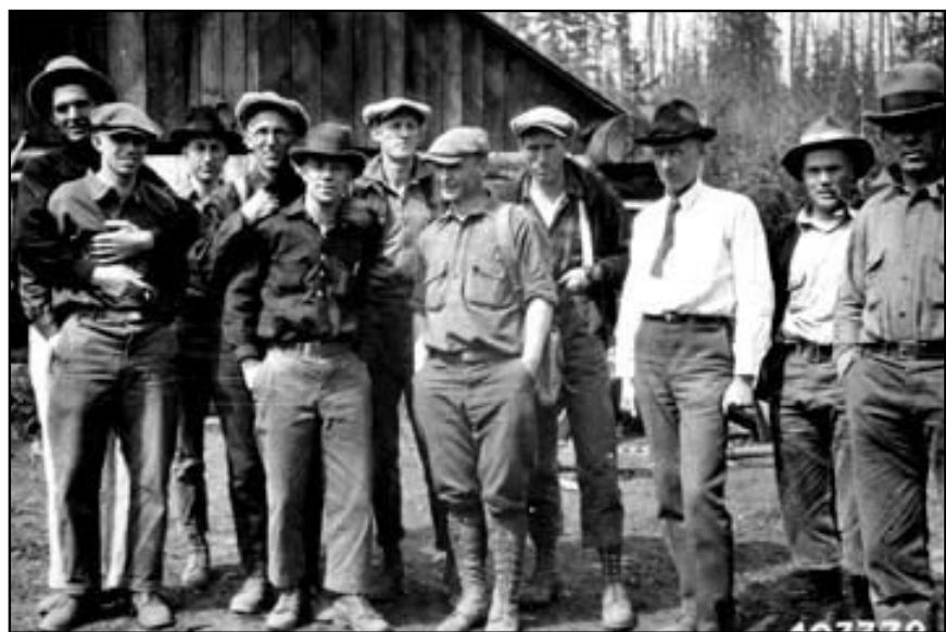
Civilian Conservation Corp workers.
